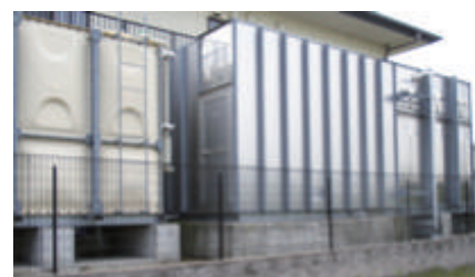
Right: Stainless Steel Bolted Type Left: FRP Bolted Type
